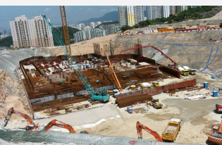
Construction of Underground Stormwater Retention Tank
