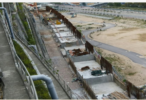
Construction of Foundation of Noise Barrier
