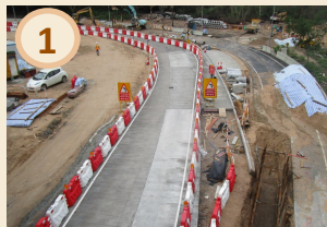
Paving road surface at slip road of Tseung Kwan O Road
